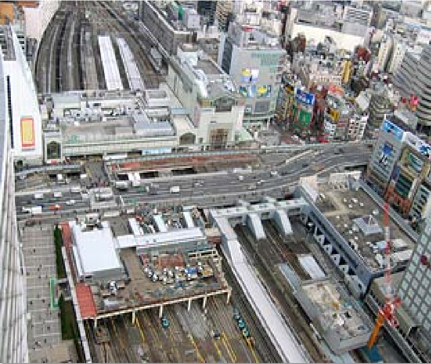
Current photo of the construction on route 20 overpass
