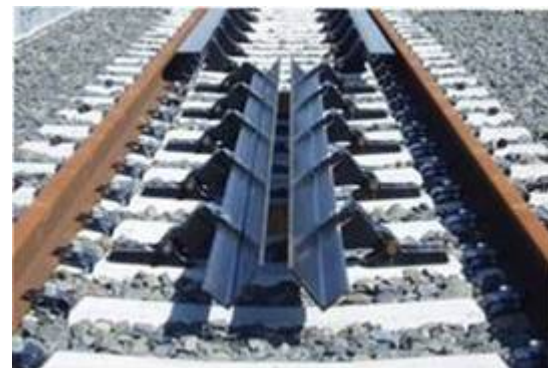
Turned over rails for track maintenance work
